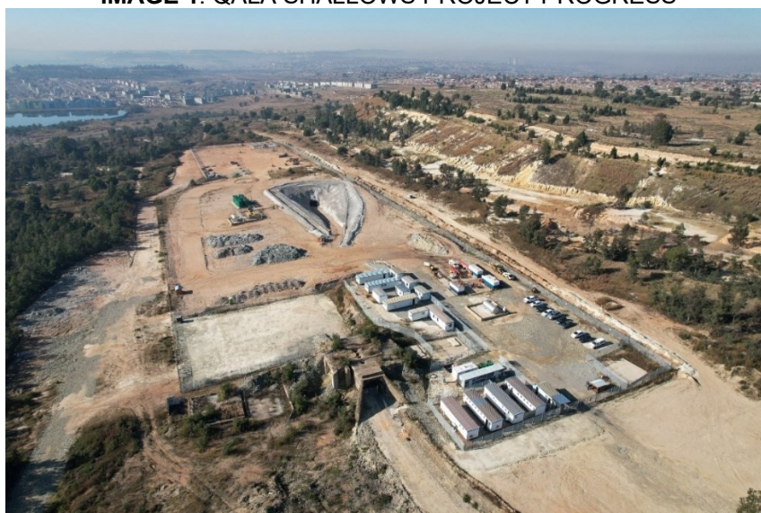
IMAGE 1: QALA SHALLOWS PROJECT PROGRESS
